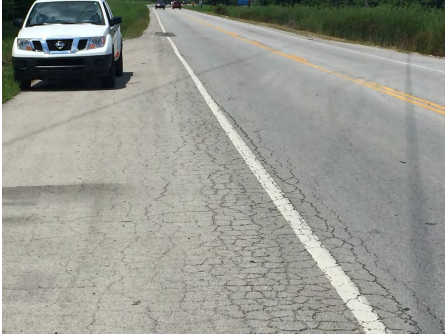
Figure 10 Alligator Cracking in flexible pavement near Metro Public Works facility
